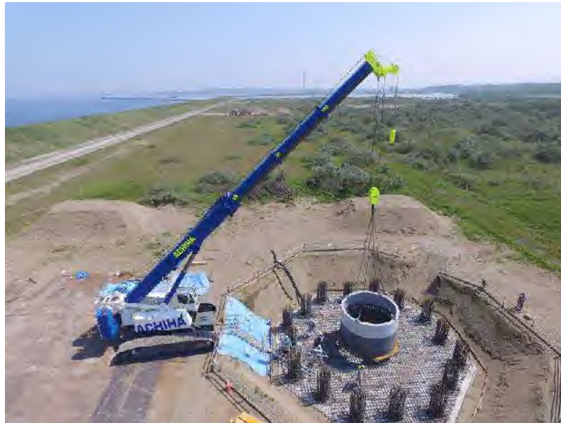
Figure 4-4-25: Anchoring Construction (Pile Foundation)
